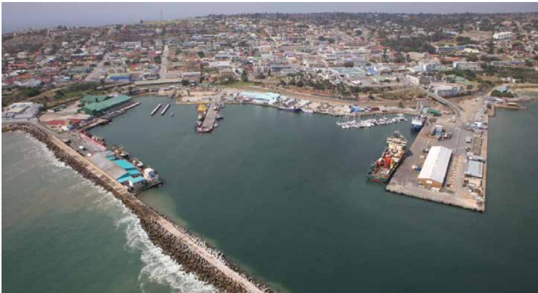
Figure 54: Port of Mossel Bay (Source: National Ports Authority)
