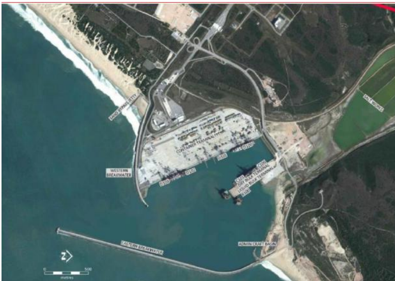
Figure 37: Port of Ngqura (Transnet Infrastructure Plans 2019)
